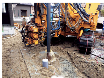
① 採熱孔掘削・鋼管建込
